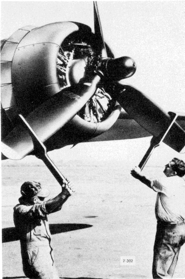
Figure 171—Changing Propeller Blade Angle
